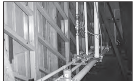
DP Air and Water Testing
